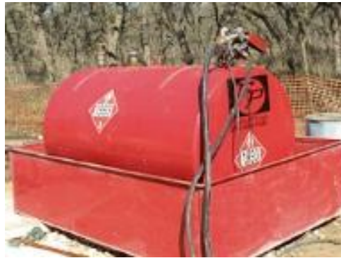
Figure 2: Metal or plastic containment pans are an inexpensive way to contain fuel or oil in case of a spill or tank rupture. It is necessary to ensure that the containment pan selected is rated for the material being stored. Properly designed and finished earthen or concrete liners are a suitable option for larger tanks.
